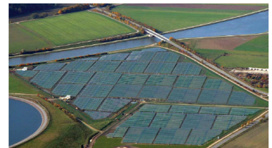
6.3 MWp, Solar Park Muhlhausen, Germany,
