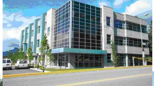
PV Buildings. Source BCIT , Burnaby, British Columbia
